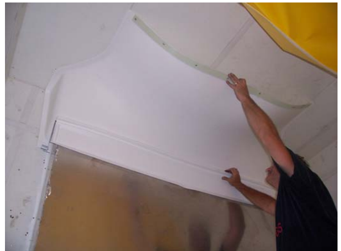
4. Hang plastic header on clips
