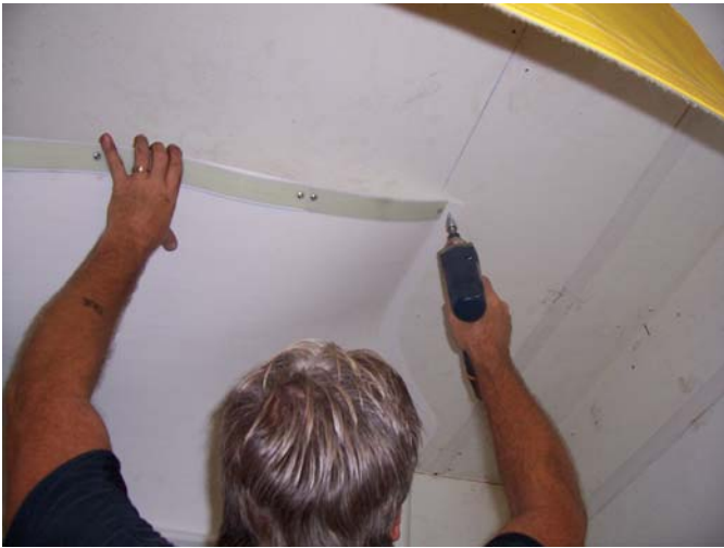
5. Screw header to ceiling
