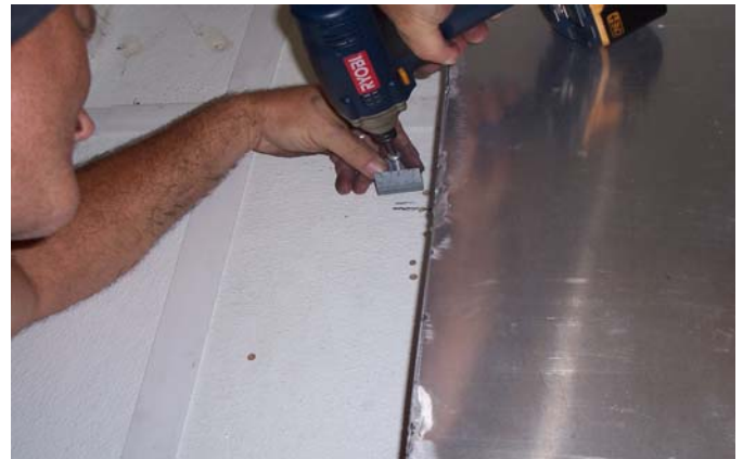
2. Install metal hanger clips
