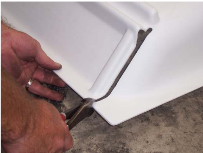
3. Cut tab for inset refer units
