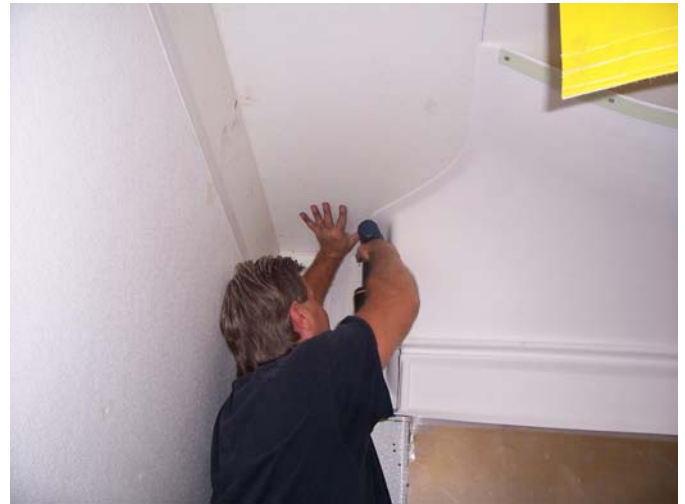
6. Screw header to side post
