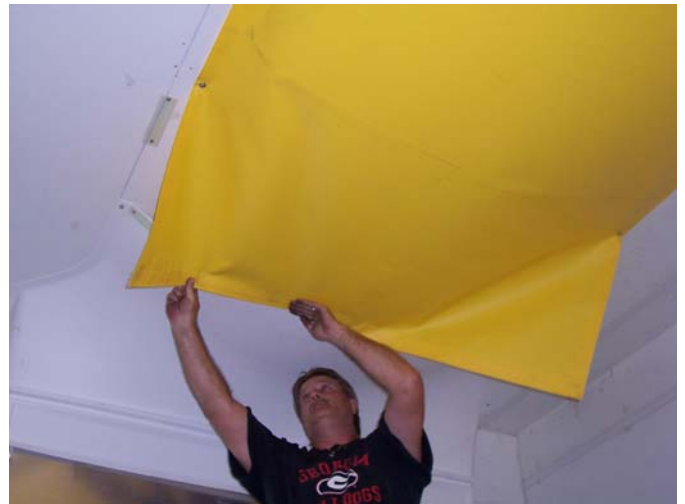
8. Attach Velcro body to header (Installation complete)
