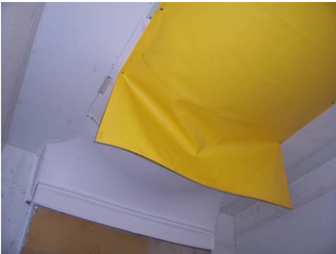
7. Install chute body
